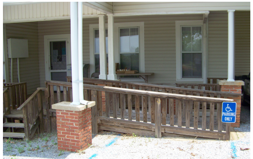
The entrance to this municipal facility does meet ADA requirements.
